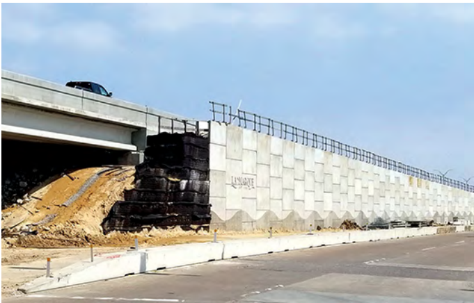
Retaining wall widening to facilitate the addition of main lanes on IH 45 near FM 1765 in the Houston District.
