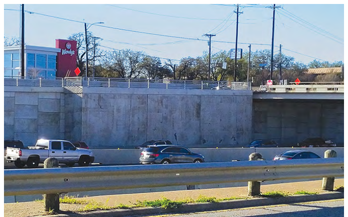
Highlighting the revised design (extended portion) of the retaining wall on TX 360 north of IH 30. This portion of the retaining wall was extended due to a change in the foundation design to mitigate a conflict with a utility duct bank.
